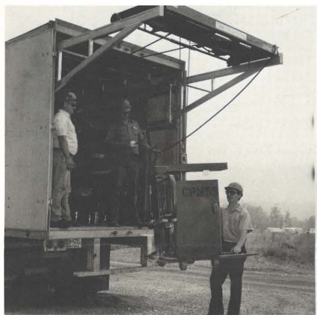
K. K. Carney, maintenance supervisor (on ground) and maintenance mechanics G. J. Korn and L. V. Parsons load individual tool boxes into the trailer. The trailer can be loaded, transported and unloaded at a new job site within a matter of hours.
