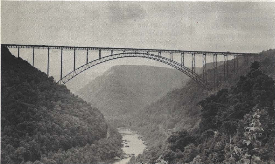
Fly ash from Kanawha River Plant was used in the grout mix for West Virginia's New River Bridge, the world's longest steel arch bridge.
