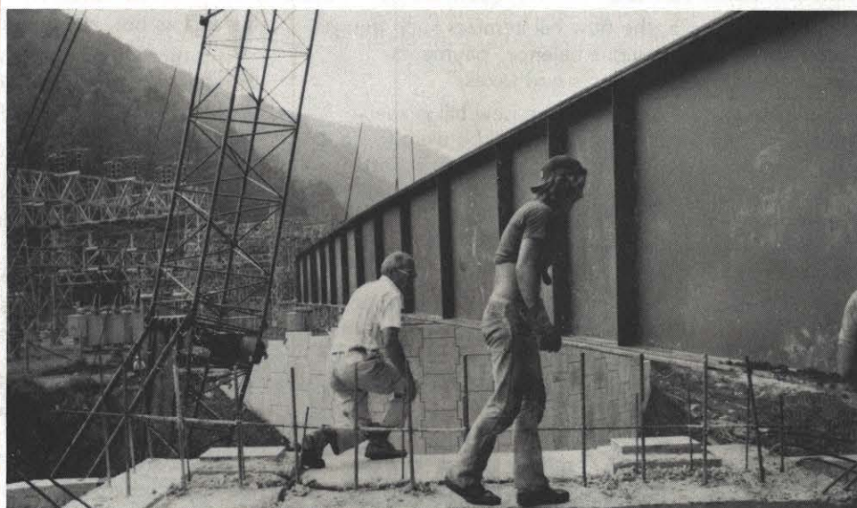
Huge crane prepares to set girder on new type of abutments.
