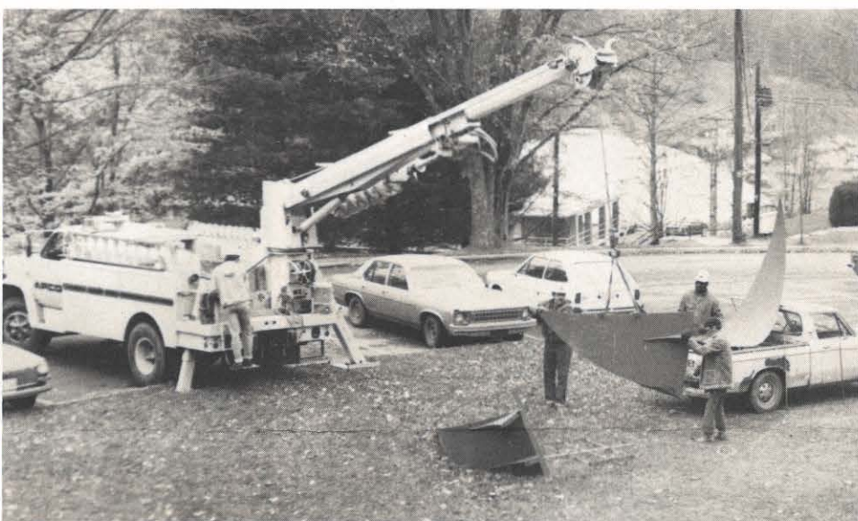
Two metal abstract sculptures were placed on the Bluefield College Campus recently, thanks to A. E. Anderson and his crew. Anderson, the father of two former Bluefield College students, supervised the unloading and placing of the sculptures, designed and constructed by Ted Guenther, a member of the Mercer County Art Guild. Guenther explained that the construction and placing of the sculptures on the college campus involved several local companies, but the sculptures would not have gotten off the ground had it not been for the use of Appalachian's crane.
