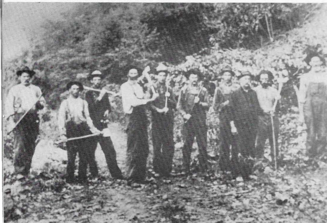
A brush cutting crew at work during the construction of Byllesby and Buck hydros.
