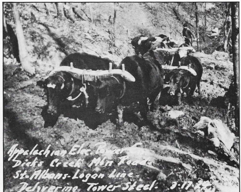
Oxen hauling steel for towers during construction of the 132 kv St. Albans-Logan line in 1924.
