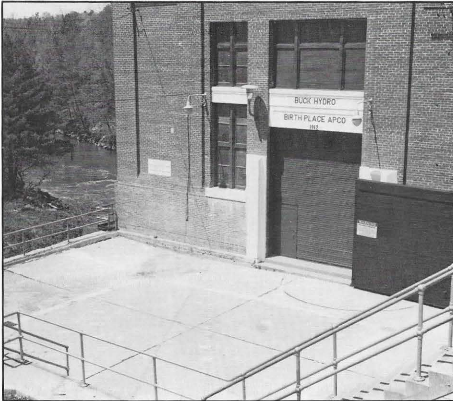
The Buck Hydroelectric Dam on New River in Virginia was one of two built by the H. M. Bylesby Company of Chicago to supply electricity to the West Virginia coal fields.
