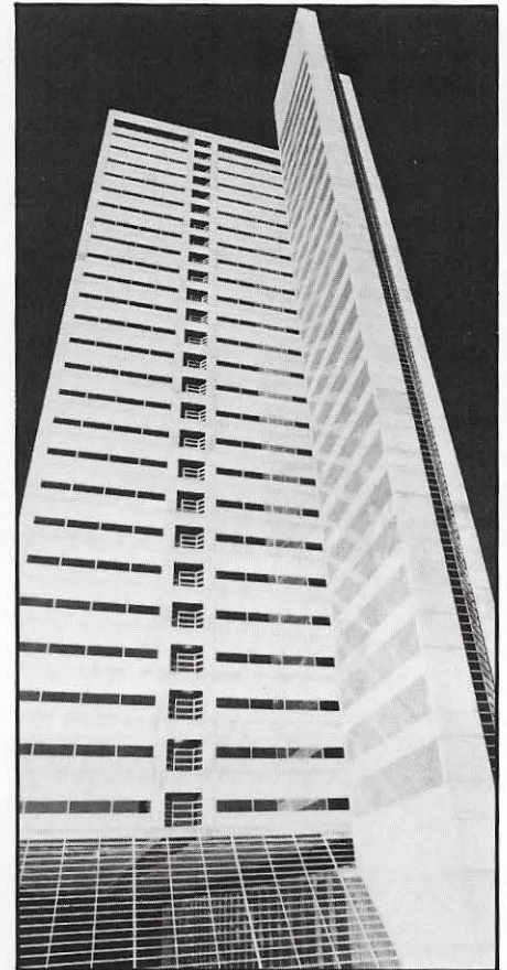
I&M's headquarters are housed in One Summit Square, Fort Wayne's new 26-story skyscraper.
