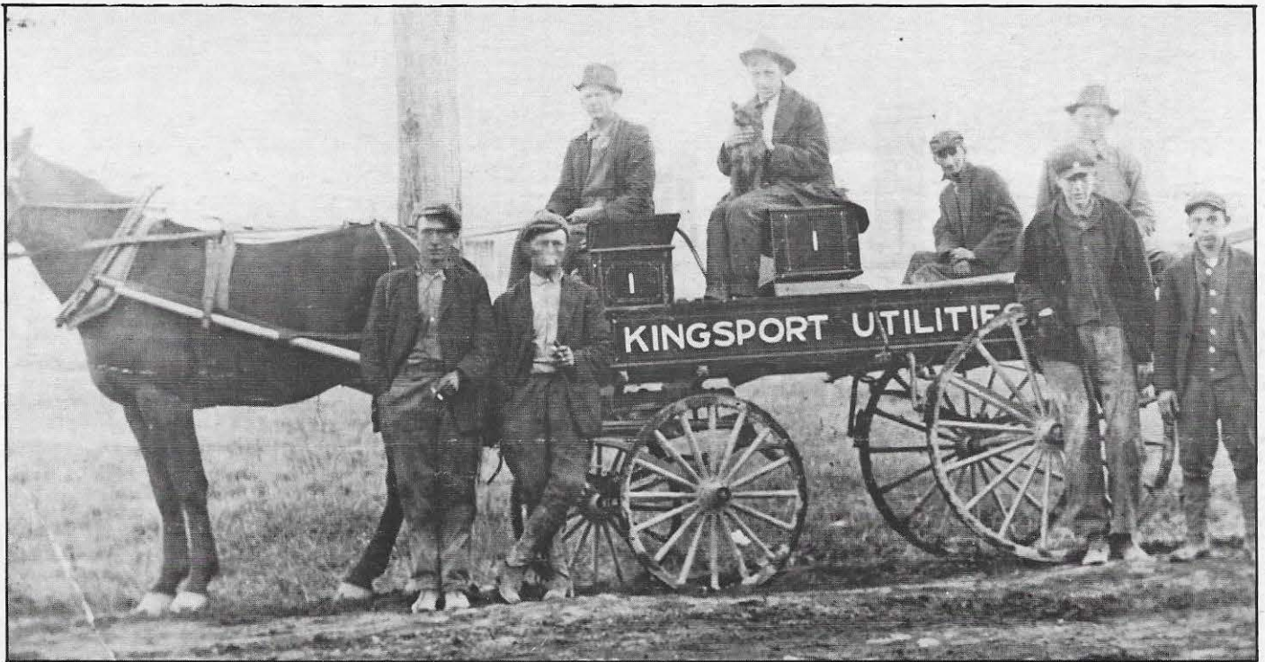
A Kingsport Utilities line crew in the early days of the company.
