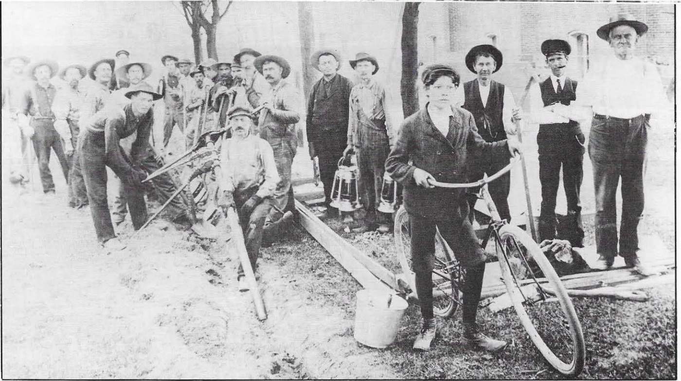
Three Rivers Gas Company employees are piping up Three Rivers for manufactured gas in 1907. The gas company was acquired by Michigan Gas and Electric Company in 1917, and the general office was moved from Ashland, Wisconsin, to Three Rivers in 1950.
