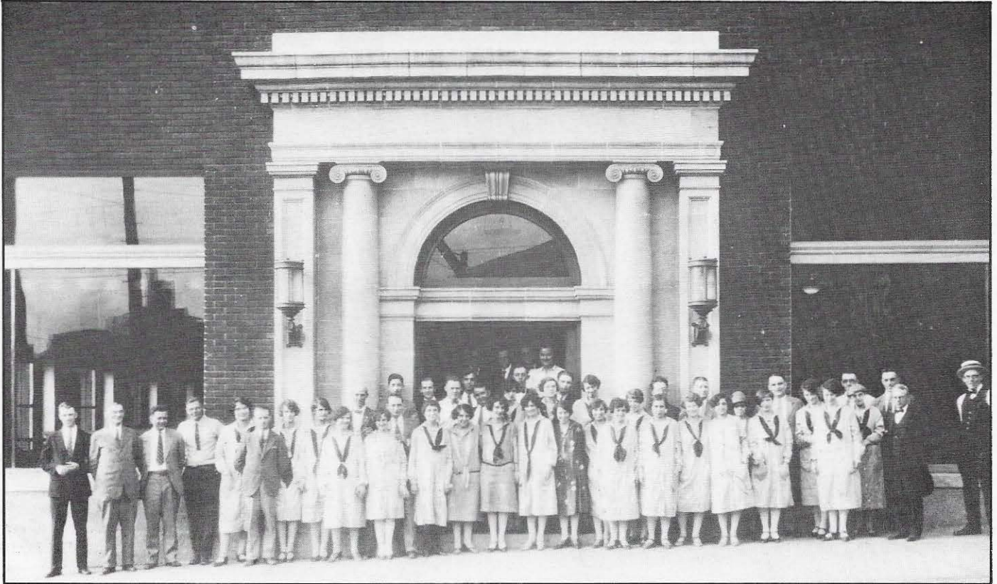
Wheeling Electric got a new look when the company occupied its new headquarters building at 51 Sixteenth Street in Wheeling in 1926, and employees wore uniforms to reflect that new look. However, the use of uniforms was discontinued after only a short time. The building remains the company's headquarters today.
