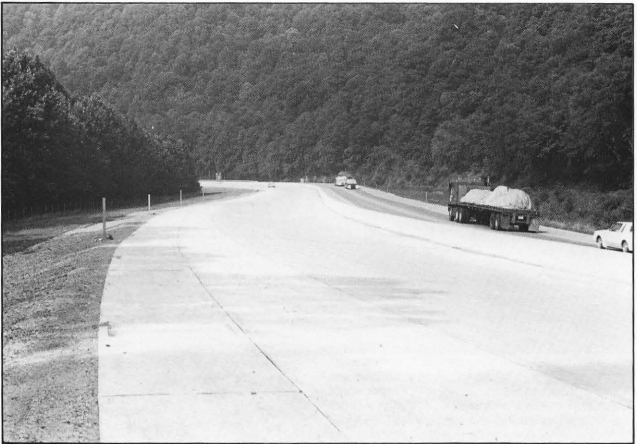
Power plant ash has been used extensively in concrete for road construction, including the roadway and median barriers on the West Virginia Turnpike. The median barriers are poured in place, thanks to the "near-zero-slump" concrete made possible partly through the use of ash in the mixture.
