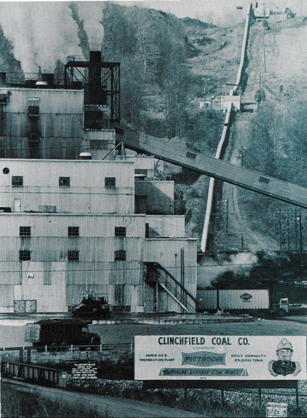
Clinchfield Coal Company's Moss No. 3 preparation plant located in Russell County. Clinchfield supplies all of the coal for Appalachian's Clinch River Plant.
