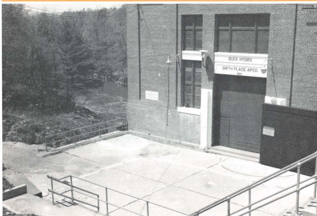
Buck Hydro, completed in August 1912, was the first of two hydros constructed on New River in Virginia by the old Appalachian Power Company.
