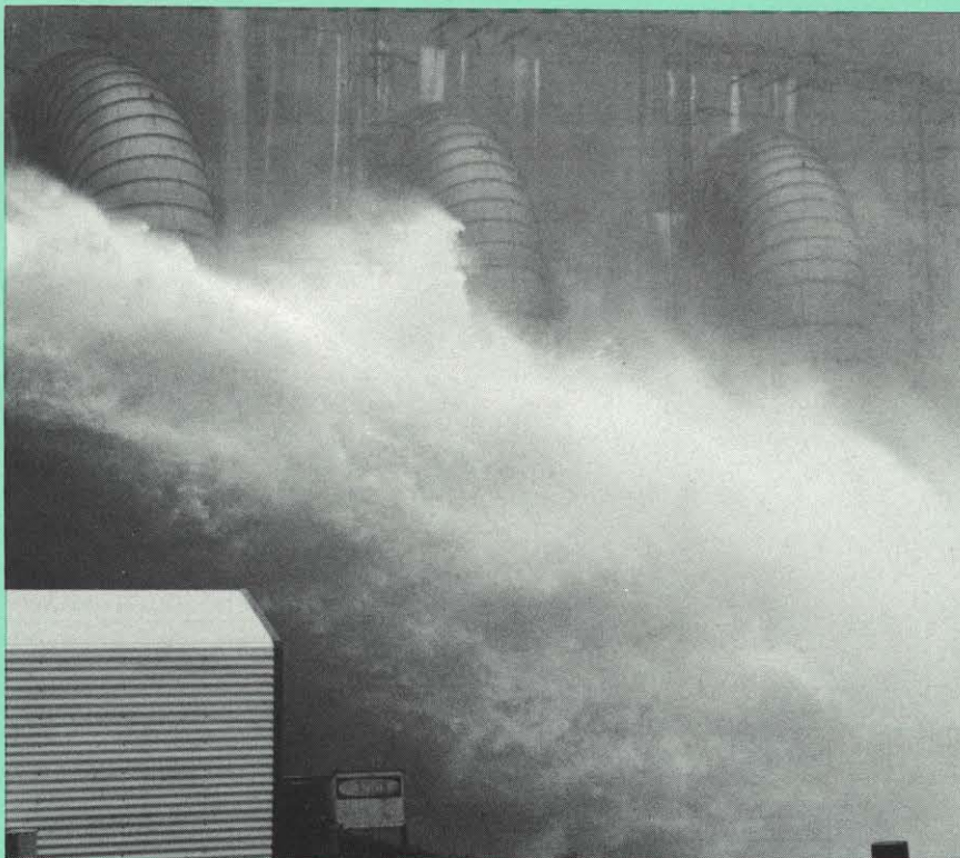
Water rushes over the spillways at Smith Mountain Dam. The GO Operations employees did an outstanding job in controlling flows from Smith Mountain and Leesville Lakes, preventing more severe damage from occurring.
