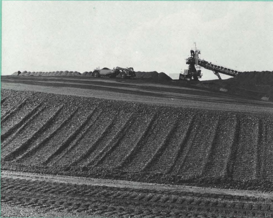
During Mountaineer Plant's 440-day record run, it burned 3.9 million tons of coal in the generation of more than 11.3 billion kilowatt-hours of electricity.
