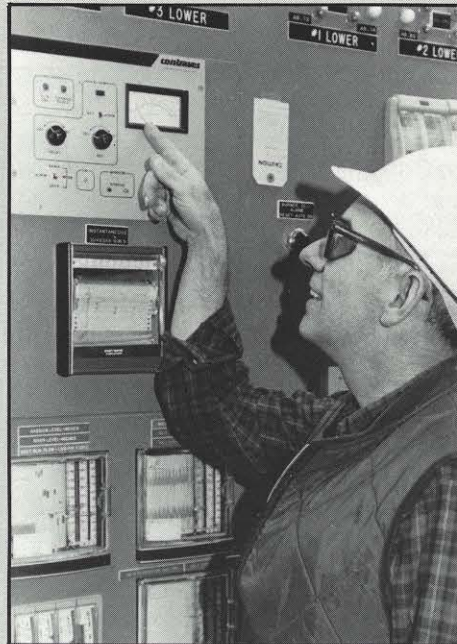
Jerry Perry, Gavin chief chemist, notes the reading in the control room of the opacity meter. The meter continuously provides data on the stack gases.
