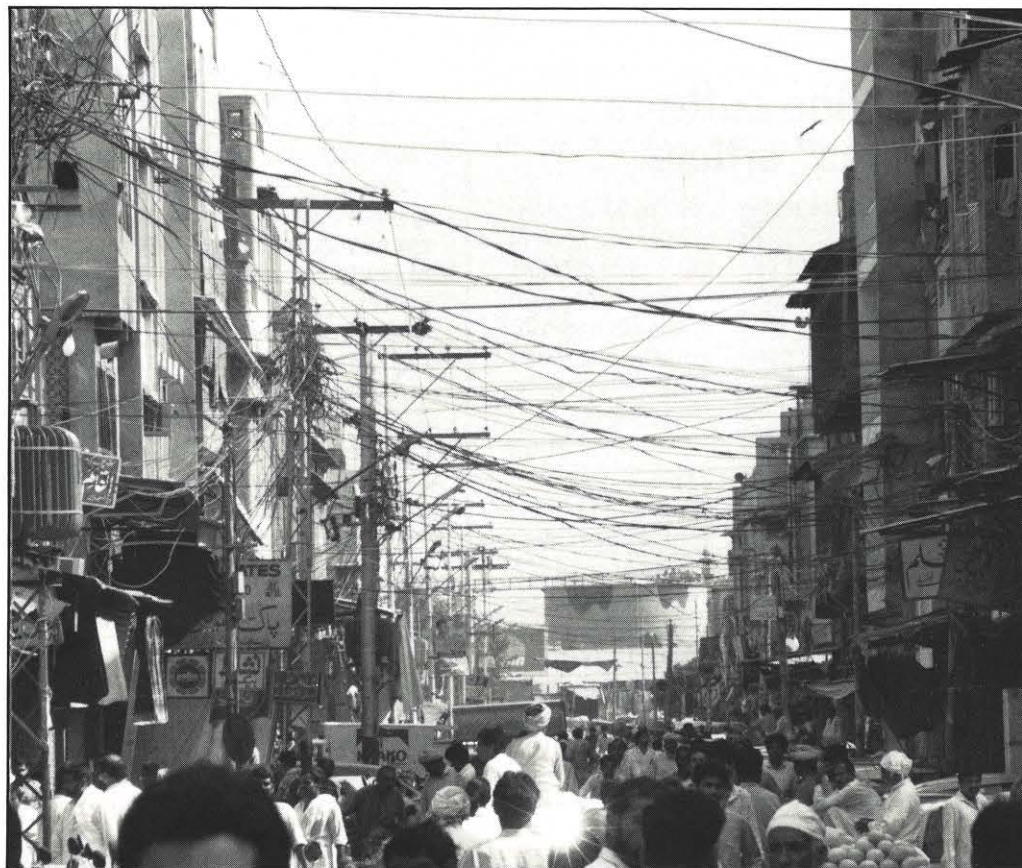
Power distribution can be a challenge in Pakistan, as this street scene in Faisalabad suggests.
