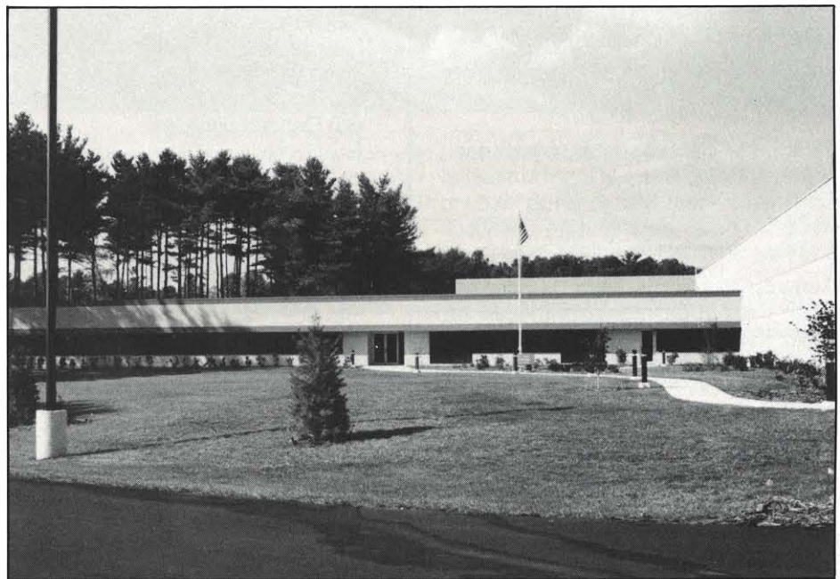
An exterior view of the new Beckley Service Center on U.S. Route 19.
