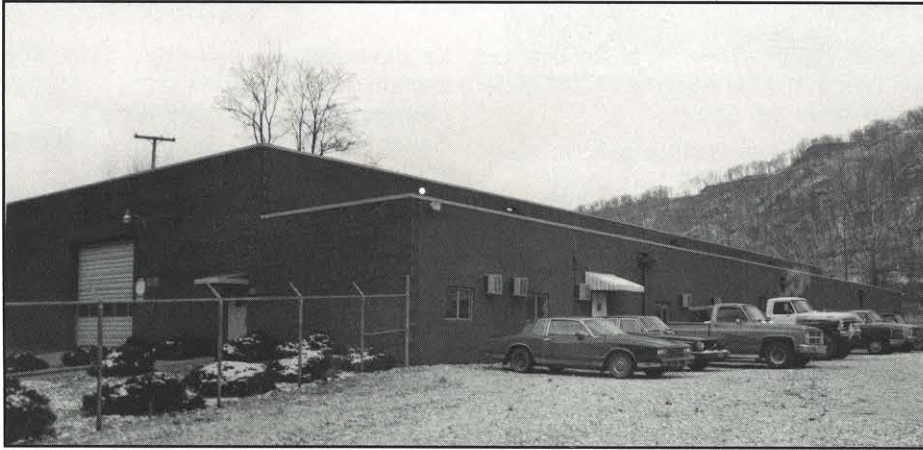
Appalachian Power has leased this facility at Hansford to serve the Montgomery operating area.
