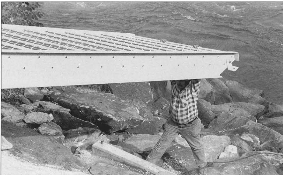
A contract workman guides a flight of steps into place.
