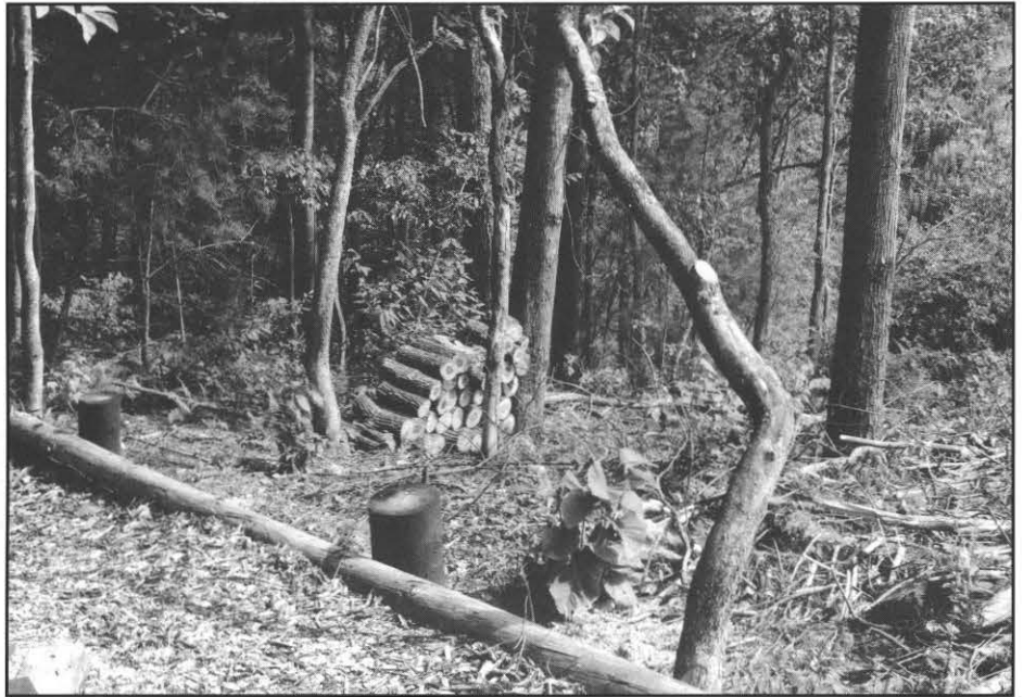
Firewood and erosion control are benefits of the vegetation management program. Brush is cut and mulched to lie as close to the ground as possible.
