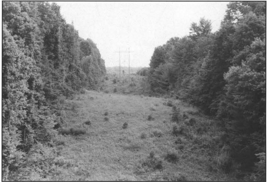
Right-of-way edge effect enhances the wildlife habitat. The trees on the left were maintained with an aerial saw; trees on the right are non-maintained.
