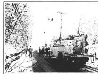
APCO crews diligently battle poor conditions to restore electricity.
