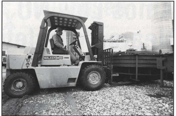
New burner registers are delivered for installation at Amos Plant's Unit 1. The register regulates the air flow available during the burning process.
