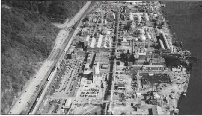
DuPont's most notable plant served by AEP is its agri-chemical facility at Belle, W. Va., in Appalachian Power's service territory.
