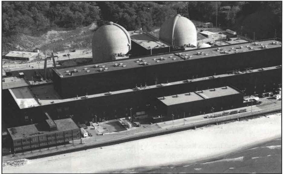
Cook Nuclear Plant's two generating units are scheduled to be operating throughout the relocation period.
